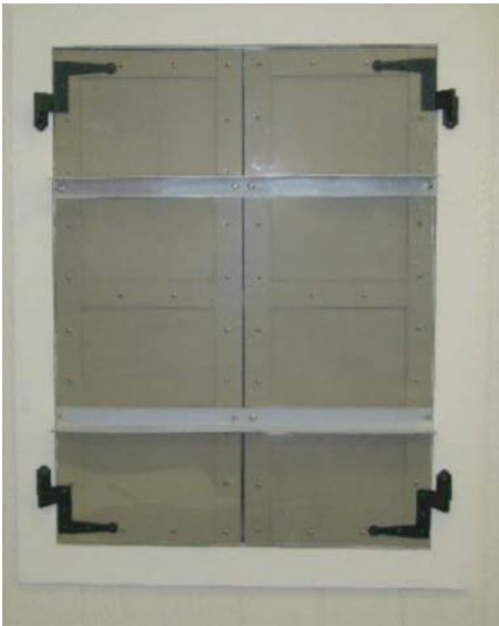
Two Storm Bars
